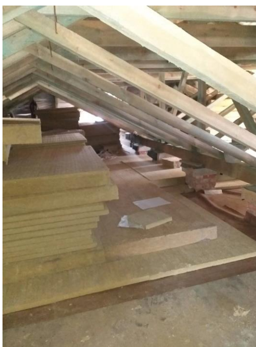
Fig. 3. Insulation of the roof of the administrative building
